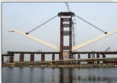
Jacking with high capacity precision control
