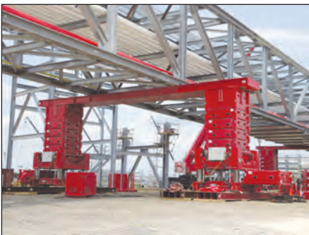
▼ Lifting an oil and gas pipe module
