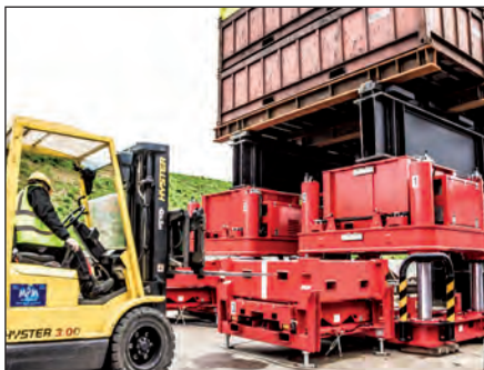
▼ A load is lifted in increments as barrels are slid into the system, lifted, and stacked; forming 'lifting towers'.
