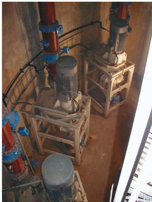
NPW 300/530 V1 newly installed in a Steel Works for Sinter Waters
